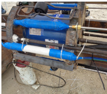
O-Cell with attached instrumentation
